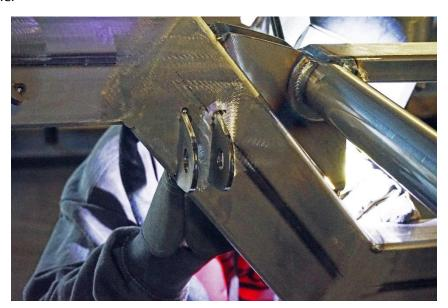
**Step 11:** Screw in the Heim Rod Ends into the Panhard bar and attached one end to the D-Tabs you just tacked in place. Now take the Panhard Bracket locate the bracket on the rear end.
